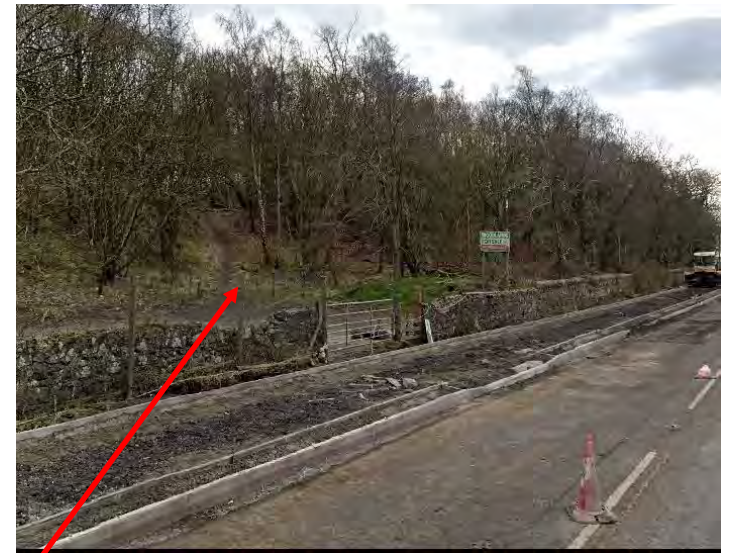
Google Streetview image (March 2021) B981 - Google Maps showing overgrown track leading to quarry from entrance.
