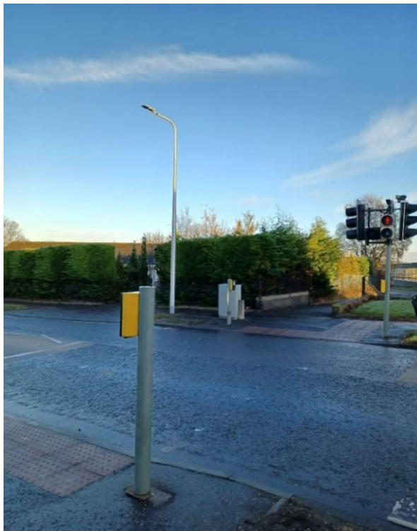
Pelican Crossing, Linburn Road
