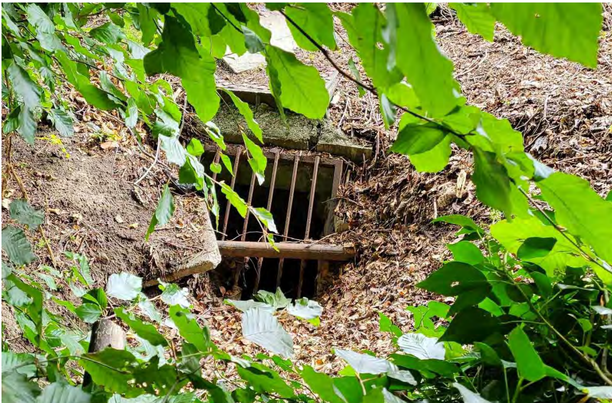
Photo 6: Culvert Inlet on Burn 1 showing debris and trash-screen
