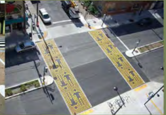
Pedestrian priority at controlled crossings
