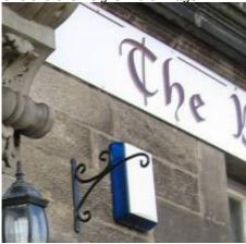
A sign screwed onto ashlar; the alarm box is insensitively placed on the front elevation – a side location would be better.
