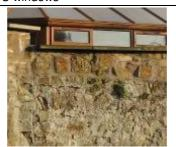
Concrete cope to rubble wall; cement pointing and unsympathetic repair
