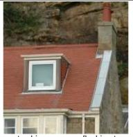
Concrete chimney cope; flashing to stone skew; synthetic roofing tiles; flat roof dormer of unsympathetic design; uPVC windows
