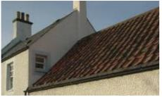
Murray House, Ramsay Lane: Outhouse roof with pantiles and slate easing. Main house: slate with open verge to the gable – unusual in Limekilns.
