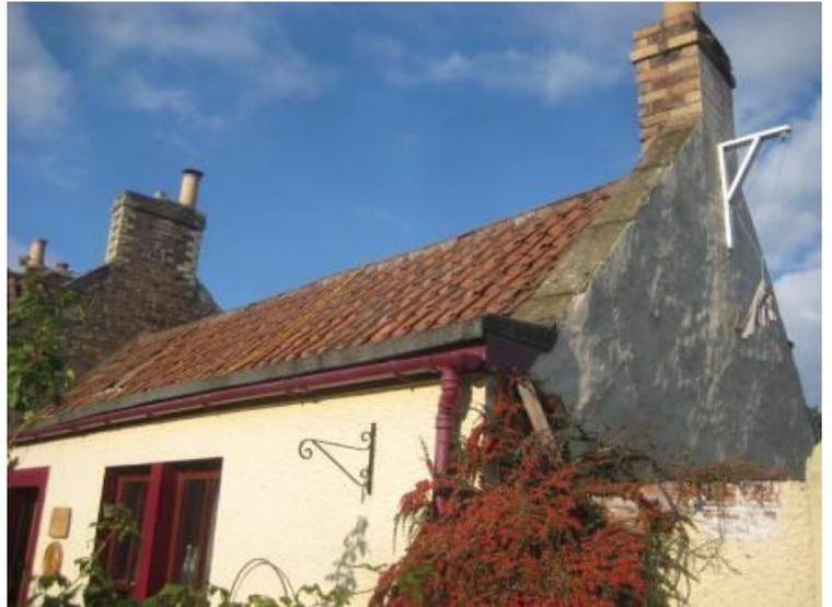
Unusual non-traditional detailing of front wall-head. A slate easing course would have been the local vernacular response to the need to improve the weatherproofing of this vulnerable area.
