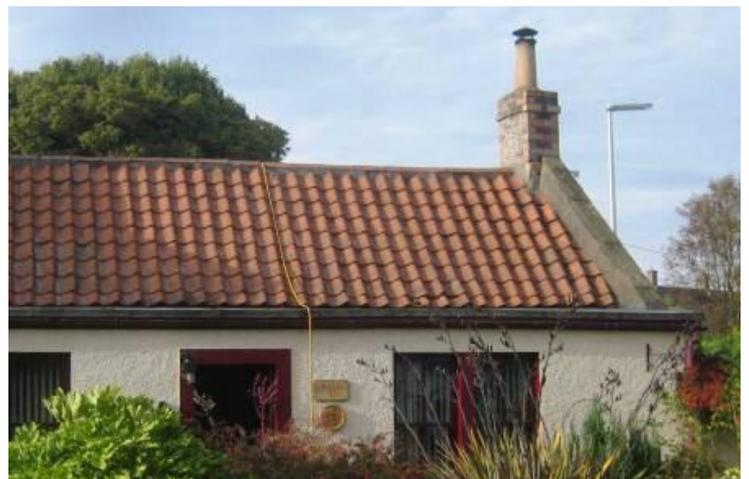
Non-traditional treatment of wallhead using lead capping.
