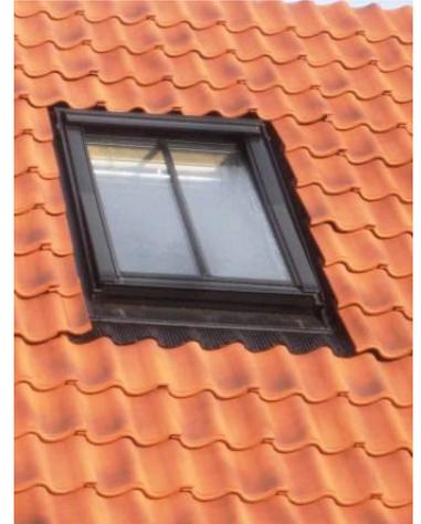
The basic design of the rooflight above right is similar to the traditional example above left. However, it is approx. 2.5 times as wide; with a dominant frame; and non-traditional apron material.
