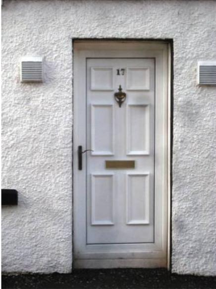
Example above: design, colour, materials and detailing including door furniture all inappropriate for a building of this period and type.
