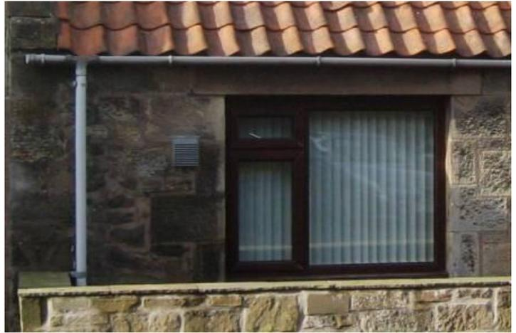
Enlarged window opening; stained dark wood frame; PVCu rainwater goods; new boundary wall with narrow cope; cement mortar pointing; vent grill.
