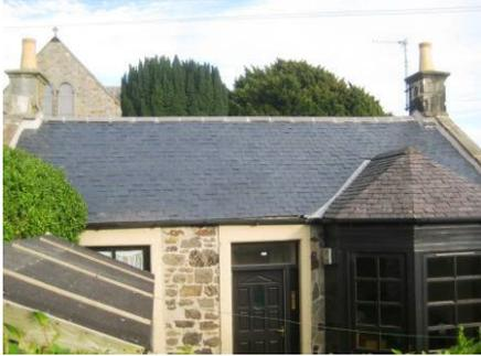
18 Schoolhill above originally would have been like adjacent 20 Schoolhill (below). Now has new roof slates and ridge tiles (was pantiled); inappropriate door and window style, colour and material; bay window added.
