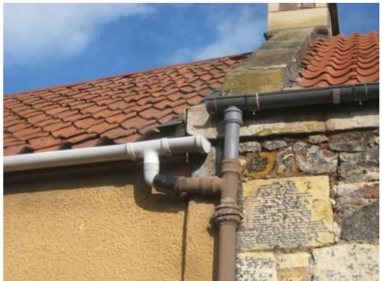
Mixture of materials, finishes and profiles used for rainwater goods
