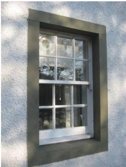
Inappropriate detailing. Imitation old Crown glass glazing in modern development. Note also non-traditional top sash horns.
