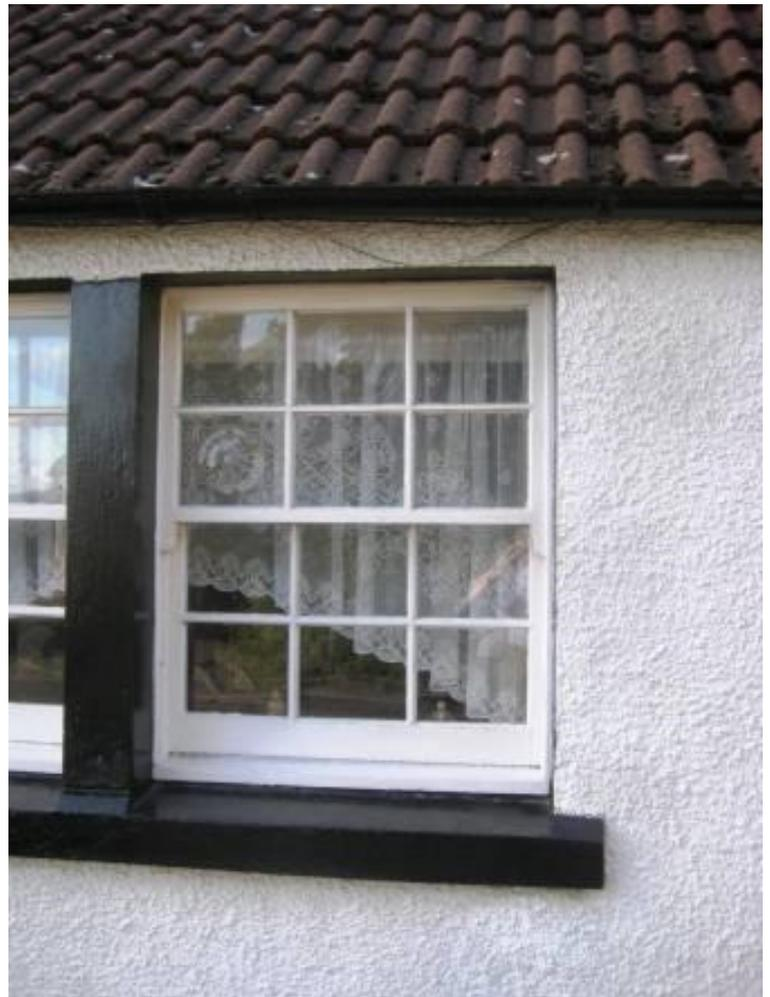
Example above: window detailing of 'horns', sill depth and crown glass all inappropriate for a building of this period and type.
