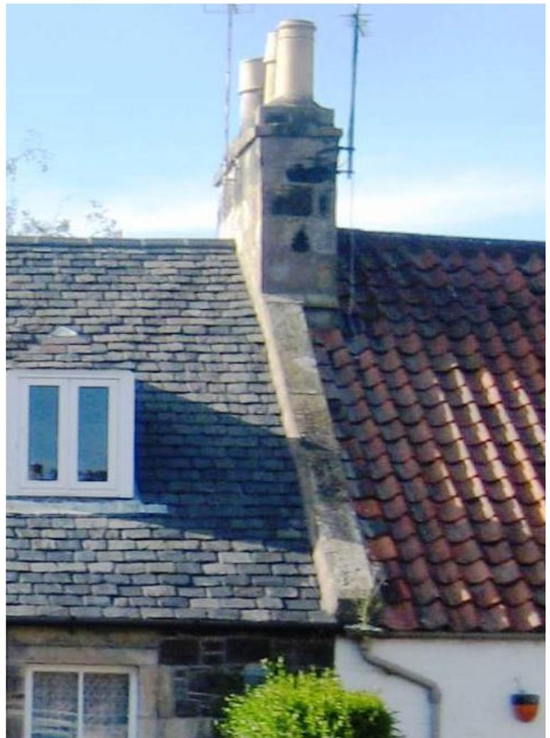
Characteristic features of Fife vernacular architecture – raised gable wall heads and red clay pantiles. Note: thackstane chimney head detail and 'blue' slates.
