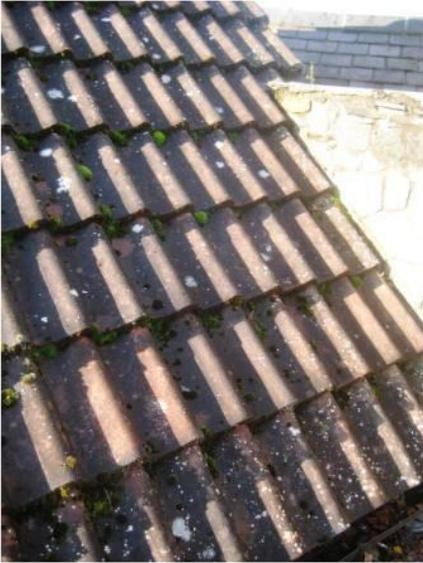
An example of inappropriate concrete roof tiles used on a building in the conservation area.
