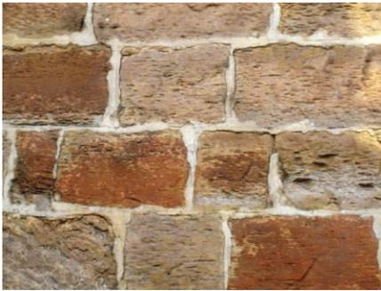
Example above of the adverse effect of cement mortar on masonry.
