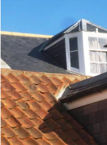
Above - synthetic fibre-cement roof slates used on a late 19<sup>th</sup> century category B listed building.
