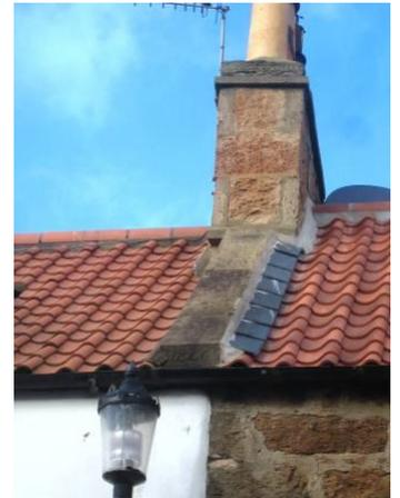
Examples of non-traditional skew cope detailing. Left-lead sheet encasing the gable skew cope. Right-row of slates over tile /skew junction.
