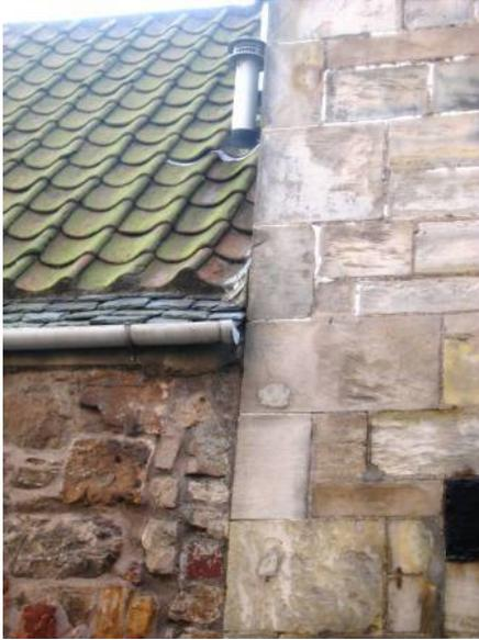
Rough rubble masonry left contrasting with snecked squared rubble right with its mixture of risers, levellers and snecks. Note characteristic traditional pantile roof with a slate easing course.
