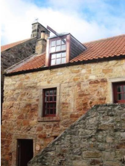
18<sup>th</sup> century category B listed house with the harl removed, and a second dormer complete with replica net hoist gantry added.
