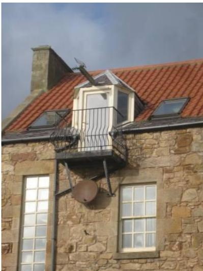
many of the 'dormers' are mid to late 19<sup>th</sup> century additions with, originally, associated hoist gantries inserted to provide access to the roof space sail lofts. Fixed external hoists were sometimes used for the nets, but sliding dormer beams were more common. Usually seen as a single central dormer per unit they were either designed as part of new houses or added to earlier ones during the mid-19<sup>th</sup> century herring fishing boom.
