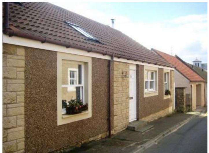
Traditional cottage with imitation stone cladding, dry-dash render, enlarged windows, PVCu door, modern sky-light, concrete roof tiles.
