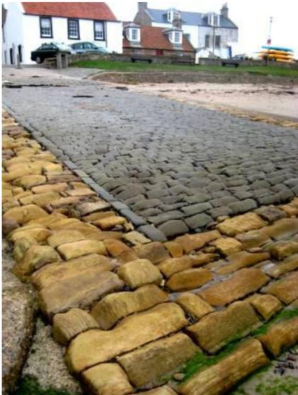
Harbour slipway constructed of whin sets with sandstone margin.
