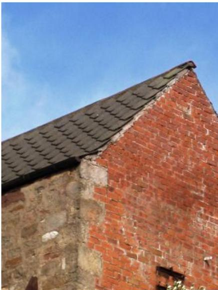
Category C listed 19<sup>th</sup> century store with brick rear gable wall. One roof slope has had the pantiles replaced since listing with modern grey concrete tiles.
