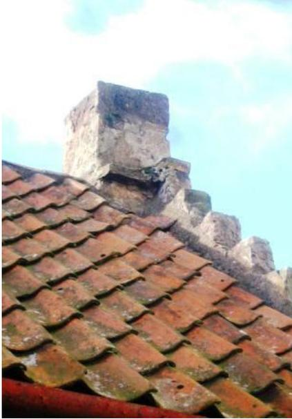
Example of a thackstone detail at base of chimney head
