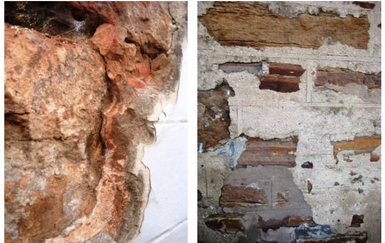
Above examples of the use of modern cement render on traditional sandstone rubble masonry (left) and pointing mortar (right).
