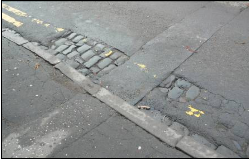
Setts on Bonnygate partially covered with blacktop
