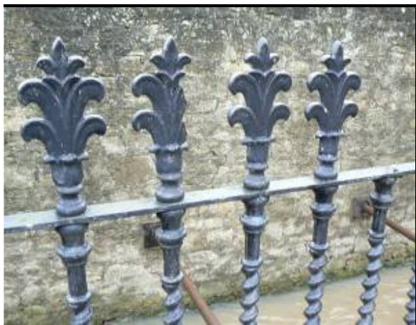
Ornamental cast & wrought iron railings on St. Catherine Street
