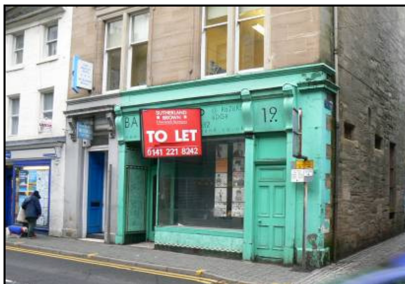
Empty shop for let – the shop front in increasingly poor condition
