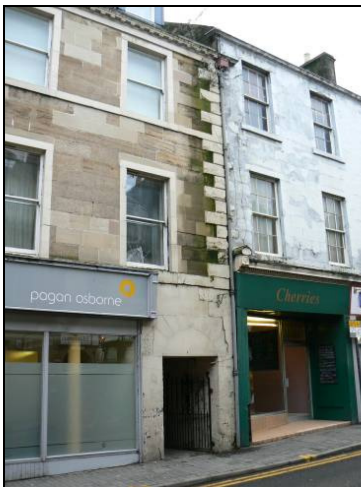
No.1 Crossgate – poor maintenance has damaged stonework on adjacent buildings
