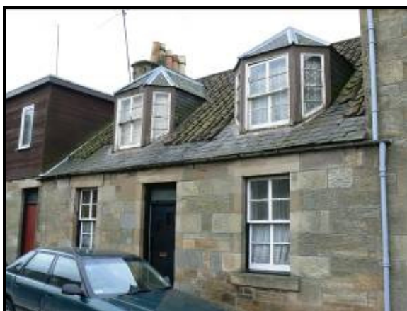
Pantile and slate roof
