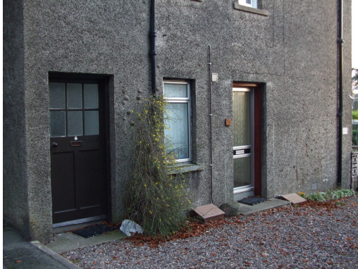
Original door and inappropriate replacement Sash and case windows in Cadham Square on the right in Cadham Terrace
