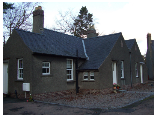
Exposed brick base course and ornamental brick at the gable in a smaller house type
