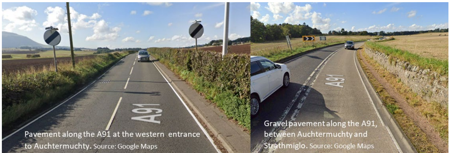
Figure A1-6: Photos showing the pavement condition along the A91.
