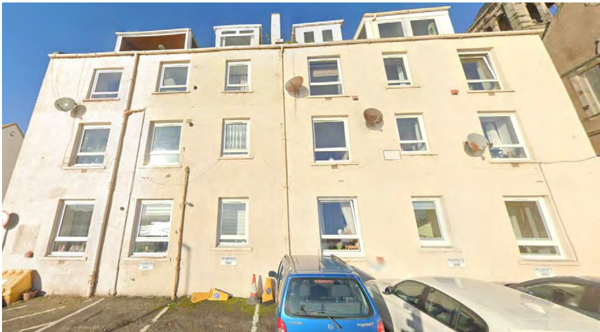
Barton Buildings, Southeast Elevation
