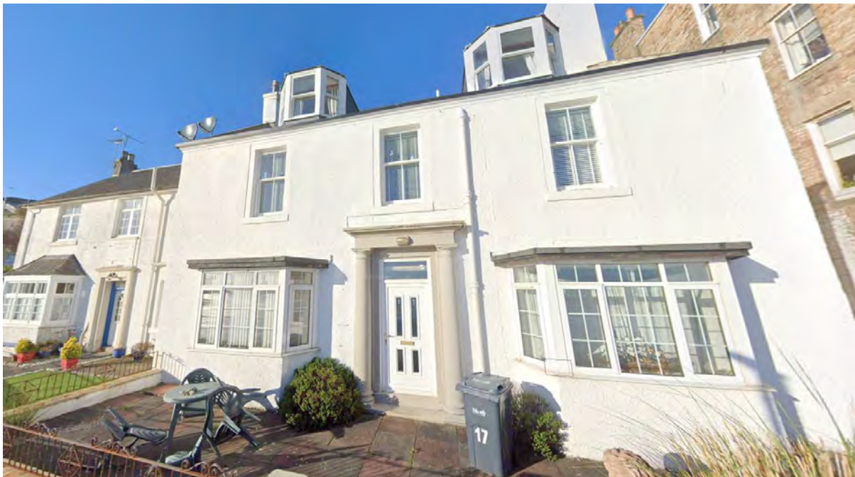
Adjacent to Providence House, Southeast Elevation
