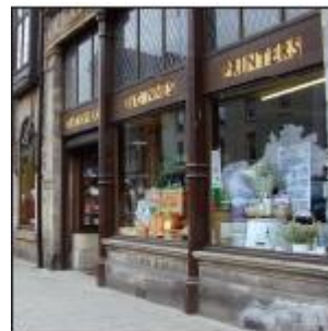
The style and scale of signs respect the building's character. The fascia is the strip on which the shop's name is displayed.
