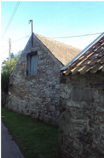
Gutterless projecting pantile roof
