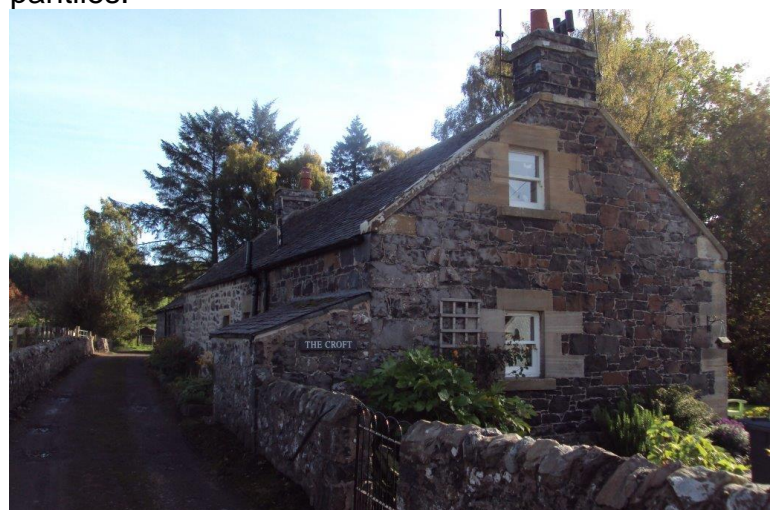
Dark rubble whin stone masonry with extensive use of pinnings, contrasting with blonde sandstone margins.
