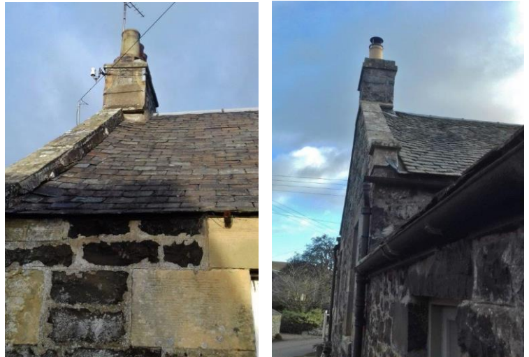
Left - cracked cement skew fillet. Right – improved lead watergate detail.
