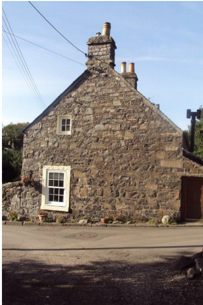
Rebuilt chimney head with retained thack stanes.
