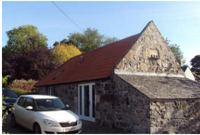
French window, vent pipes, French and roof windows and cement pointing on a listed building.
