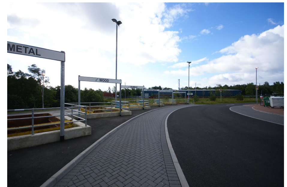
View of Skip Area & Infiltration Paving
