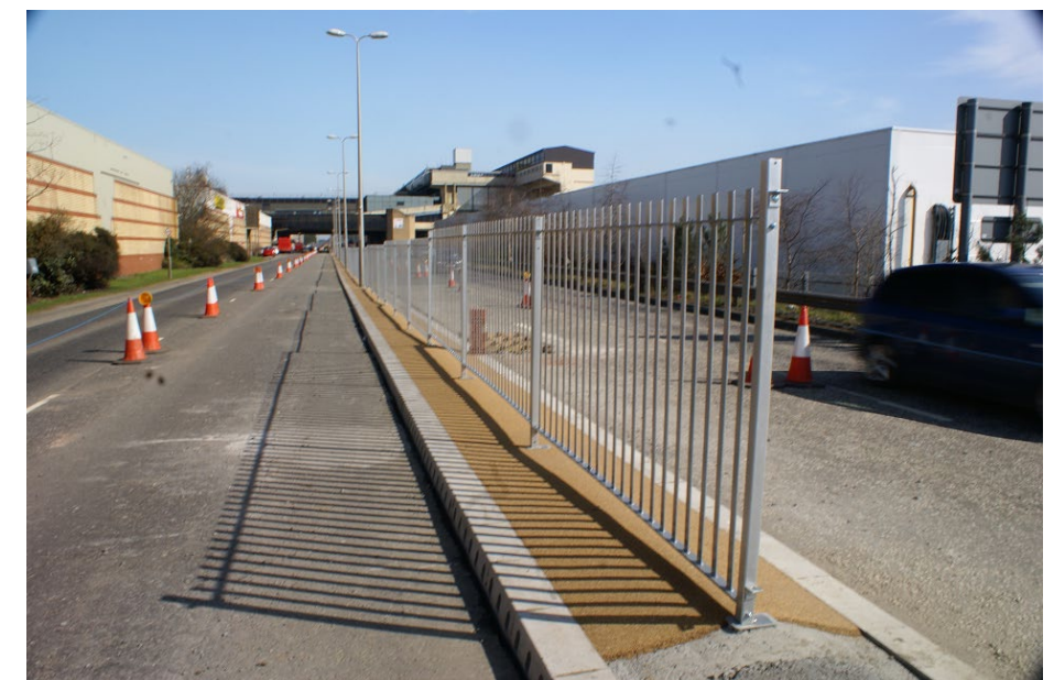
Resin bound gravel & drainage kerb
