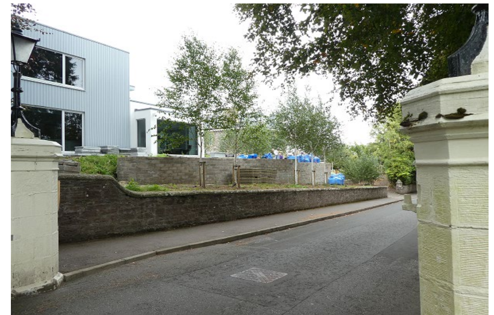
Tree planting & retaining wall
