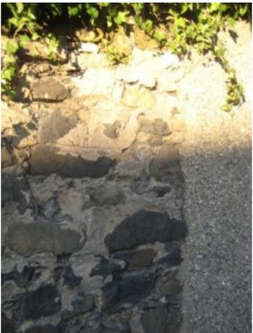
Cement mortar and dry-dash render on a wall.
