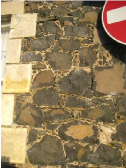
Whinstone rubble masonry with sandstone margins
