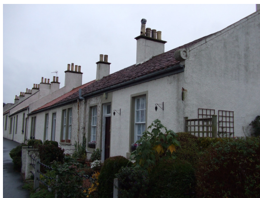
Scroll skewputts and uniformity in chimney stacks and harling/ roofing materials
