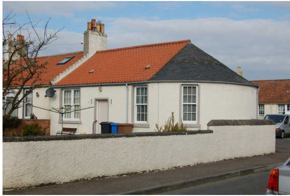
Slate used on the rounded corner of an end terrace cottage roof.
