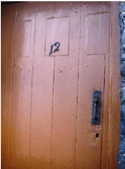
An example from within the conservation area of a style of traditional cottage door which may have been common. Note blocked former glazed panels.
