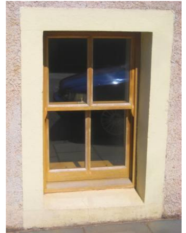
Examples of the inappropriate use of non-traditional modern varnishes on external woodwork.
