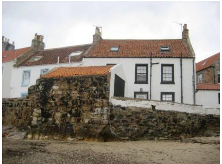
Pitch black masonry walls now painted in brilliant white modern masonry paints.
