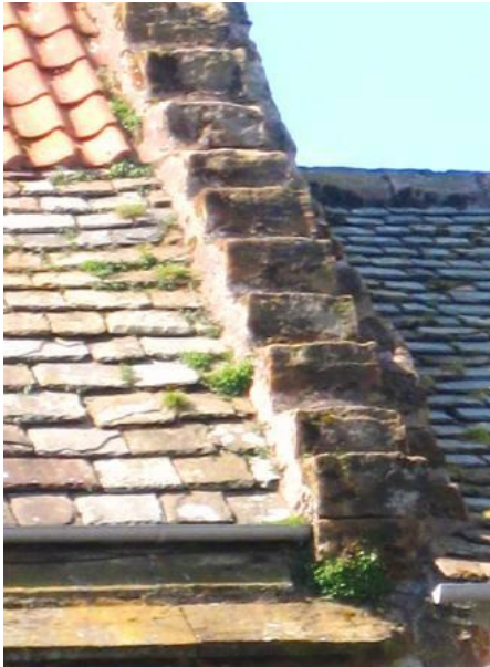
Above and below-traditional clay pantiles with slate easing course and crow-stepped gable.
