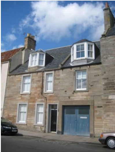
Traditional design of fishermen's houses- with ground floor workshop/sail loft and later dormer with gantry and hoist to attic floor sail store. Example below with fore-stair.
