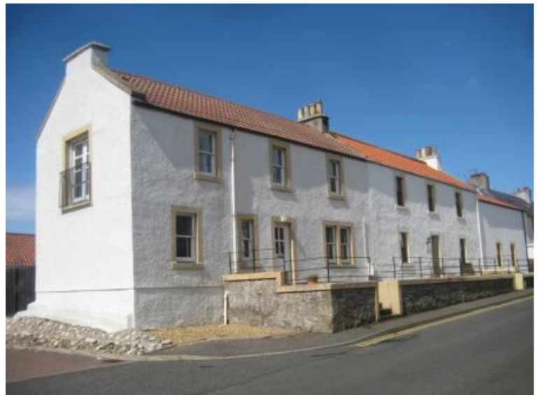
Abbey Wall Road – removal of chimney cans, capping off flue, and introduction of a balcony style gable wall window; half glazed front doors and use of brilliant white modern masonry paints gives this renovation the character of a modern development.
