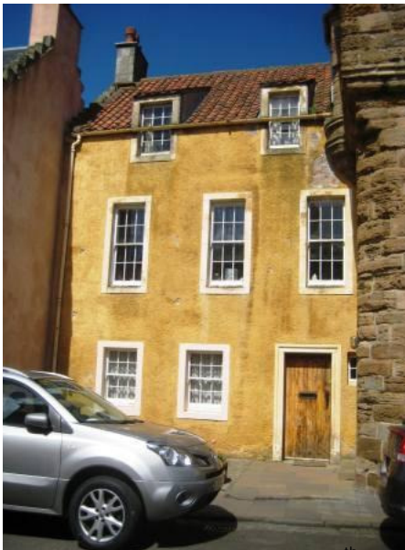
A traditional lime wash on a late 16 th century category A listed building on the High Street. The choice of an appropriate colour should be research based.
