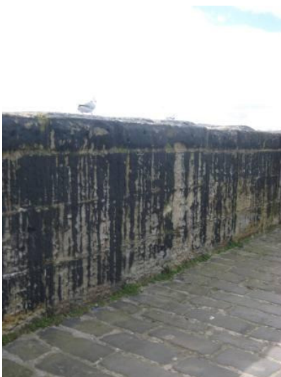
Harbour sea wall. Early form of mass poured concrete. Note shuttering lines and tar coating.
