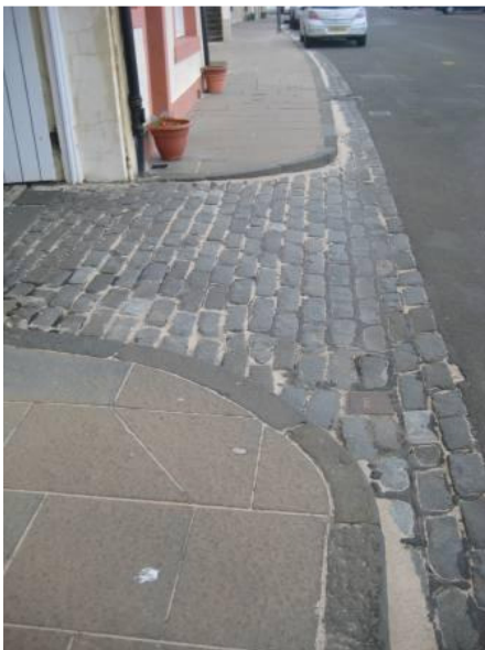
Examples of the use of original traditional whin setts and kerbstones with modern paving slabs.
