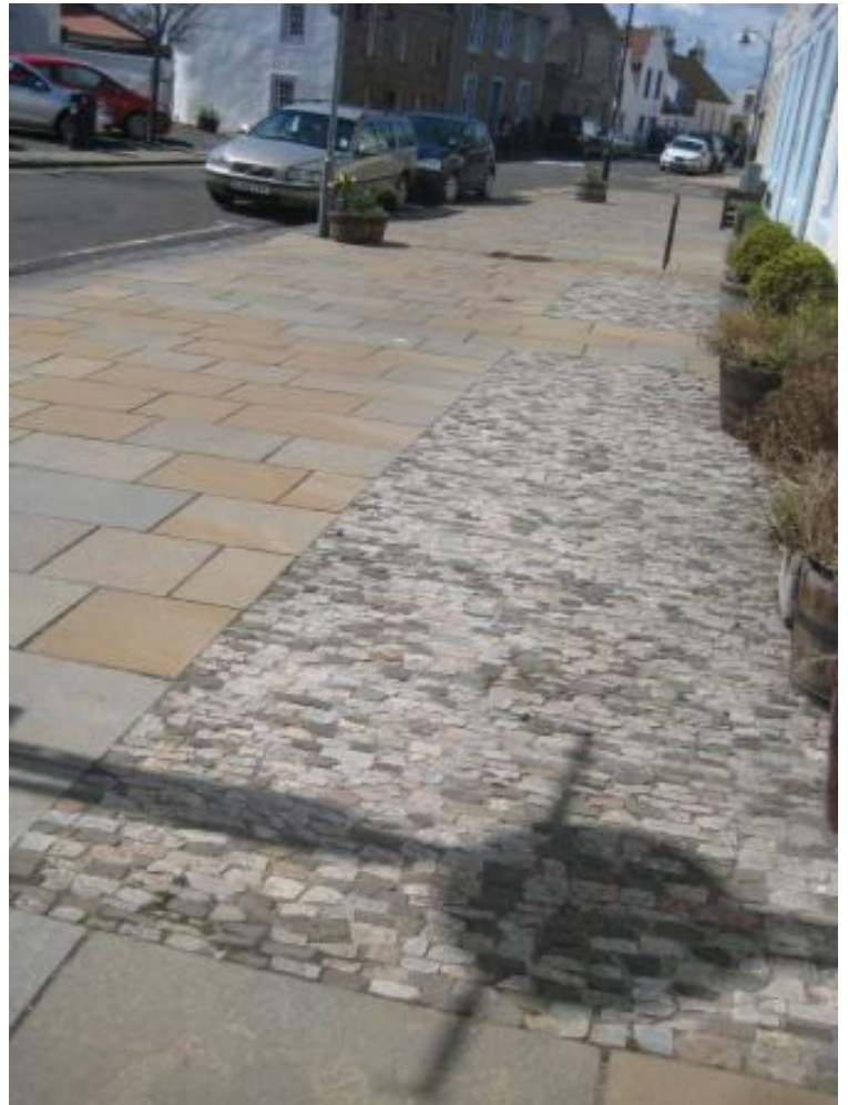
Hardscaped area on the High Street resurfaced using a mixture of paving and sudo setts/horonizing using non-indigenous stone types.
