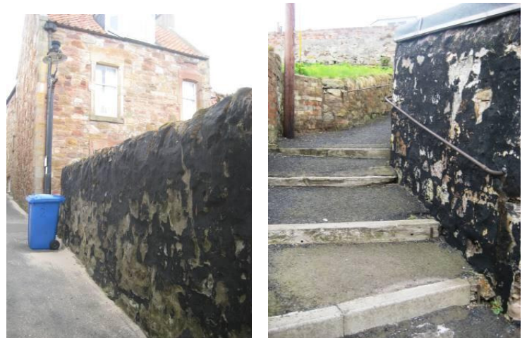
Examples of the tarred walls seen throughout the conservation area.
