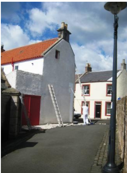
Weathered off-white mat finish masonry being re-painted with brilliant white gloss modern masonry paint.
