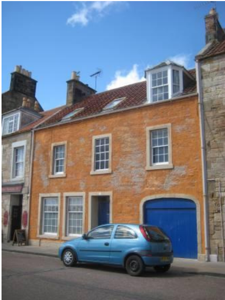
A traditional limewash in a traditional colour but inappropriate for this listed early 19 th century building on Mid Shore.
