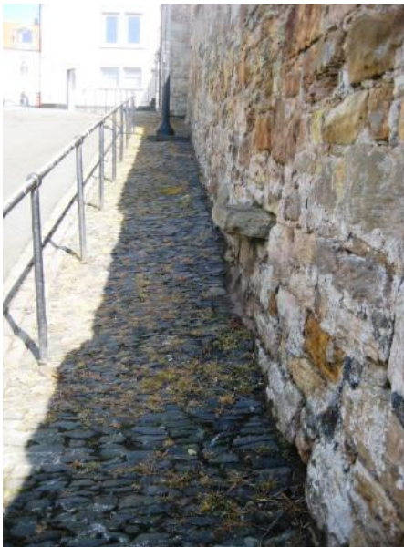
Modern resurfacing using traditional style whin horonising (Water Wynd).
