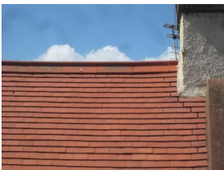
Inappropriate modern Rosemary plain roof tiles on a listed building within the conservation area.
