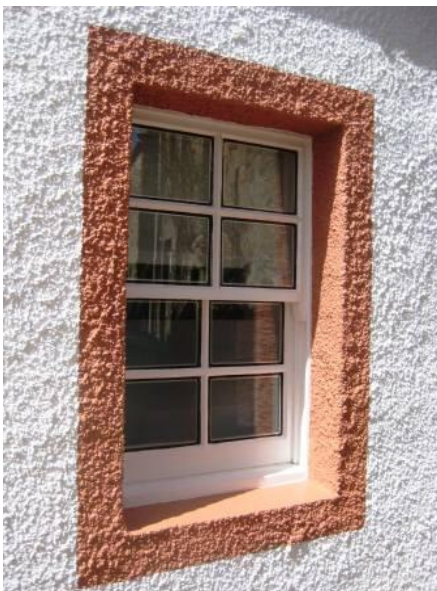
Modern wet dash render taken over window margins and a non-traditional colour scheme. Note also black double glazing strips.
