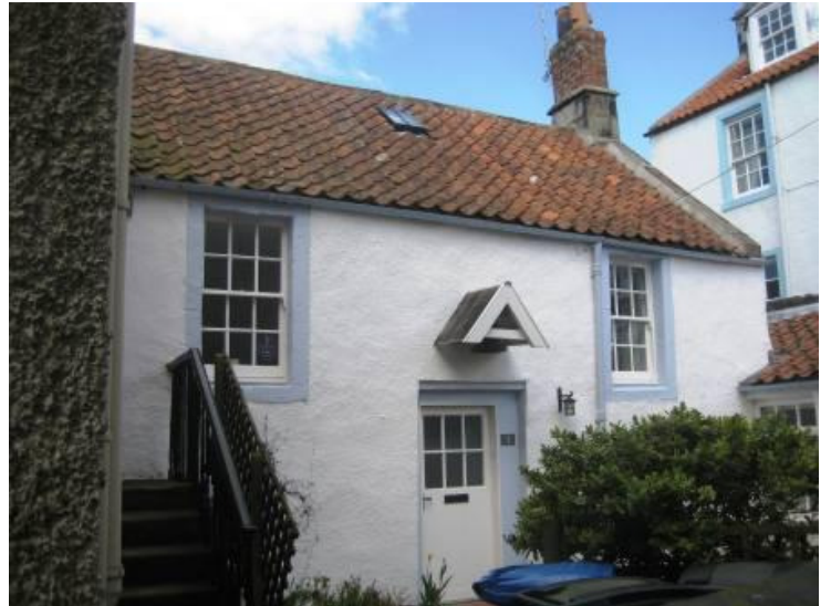
Porch canopy on a listed building in Bruce's Wynd. Note also inappropriate half glazed door and coach lamp.
