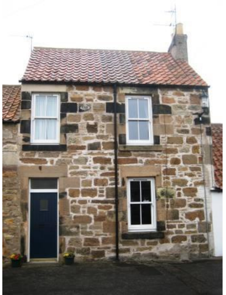
Routine Row – illustrating the negative visual impact of using modern ordinary Portland cement for re-pointing a traditional rubble masonry wall. Note also the trickle vents for the double glazed windows.
