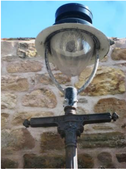
Example of the surviving late 19 th century specially made cast-iron street lamp standards now with modern lamps.
