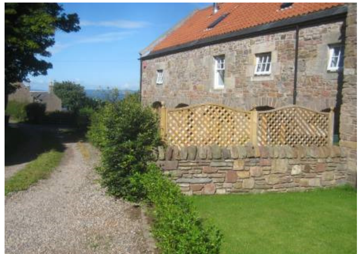
Note above: domestic style and additional windows, flue pipe and rooflights in roof; door converted to window; inappropriate modern slate easing course; rainwater downpipe; enclosed 'garden' with modern style trellis fencing and hedging. Not visible in the above are the former cart shed open bays now enclosed with heavy framed windows which read architecturally as such.
