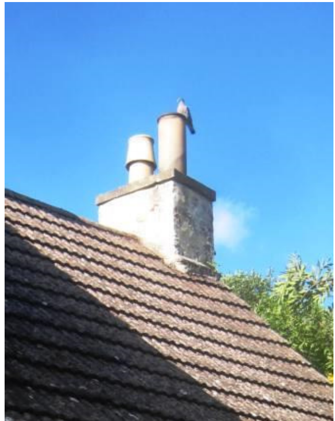
Modern concrete tiles on an 18 th century roof which may have been thatched originally.
