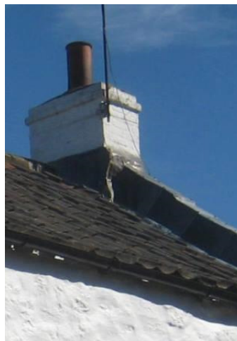
Evidence of former thatched roofs. Thackstone evident to right and steeper pitches. Ridge lowered (left) and pantiles; original pitch but later pantiles replaced with concrete tiles.
