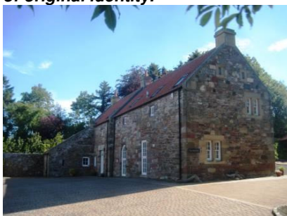
Suburban and modern features added: eaves raised; new chimney heads x3; new modern roof lights x4; doors changed to French windows; re-modelling of end bay; new windows x4 in gable wall; gable where there was probably a piend roof; chimney head; rainwater goods, etc.
