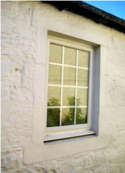
PVCu replacement of a traditional timber sash and case window on a listed building
