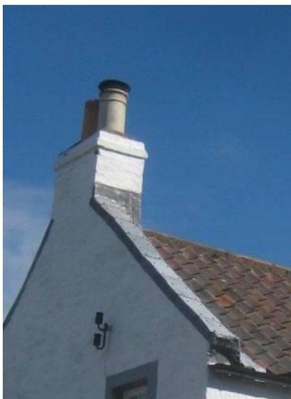
Inappropriate non-traditional detailing and use of materials at chimney head/gable (lead sheet capping).
