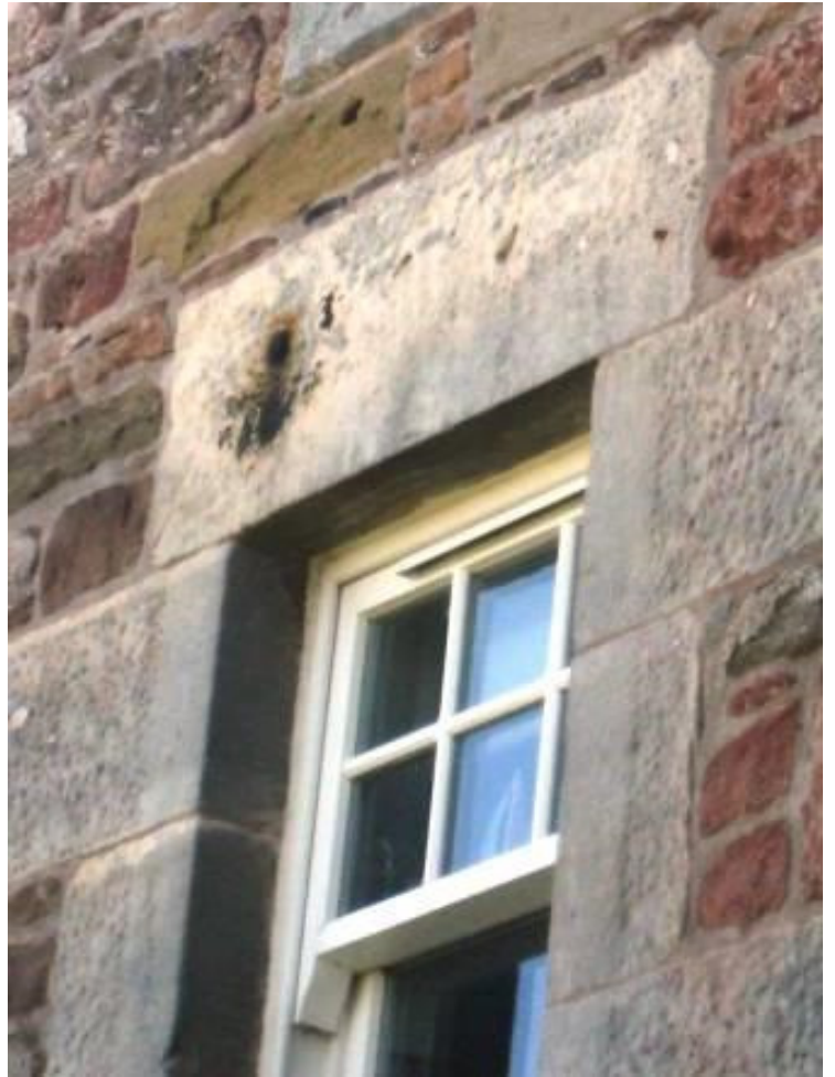
Inappropriate detailing making the above window on a listed building appear modern: trickle vent; horns; glazing beads; thicker frame; different refractive properties of double glazing.
