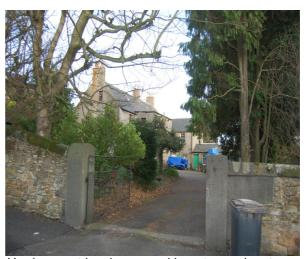
Hard cement has been used here to repair gate piers, which will cause the stonework to deteriorate over time
