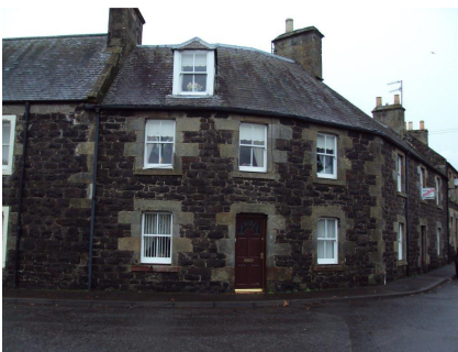
19 th century contrasting dark whin stone with blonde sandstone margins and grey slate roof.
