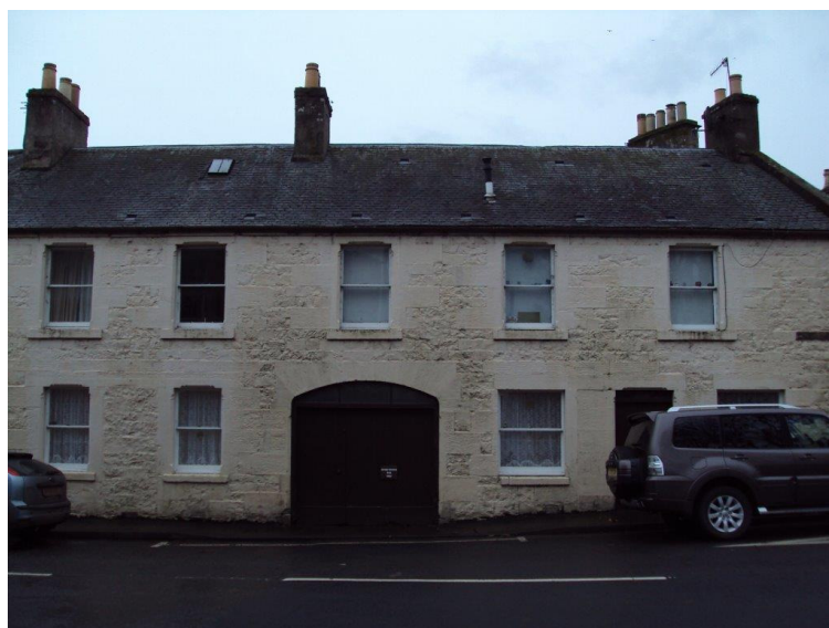
Inappropriate painted whin rubble masonry.
