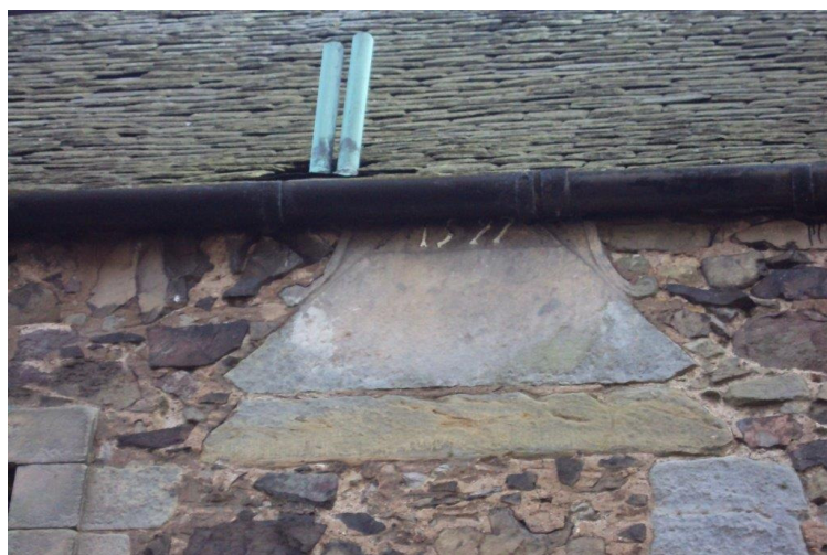
Scottish slate on Macduff House. Whin rubble masonry, probably missing an original harl.
