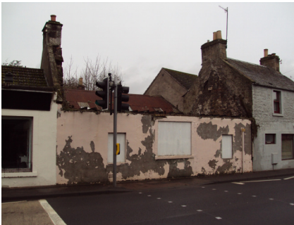
37 Cupar Road (above). Roof recently removed due to its dangerous condition.
