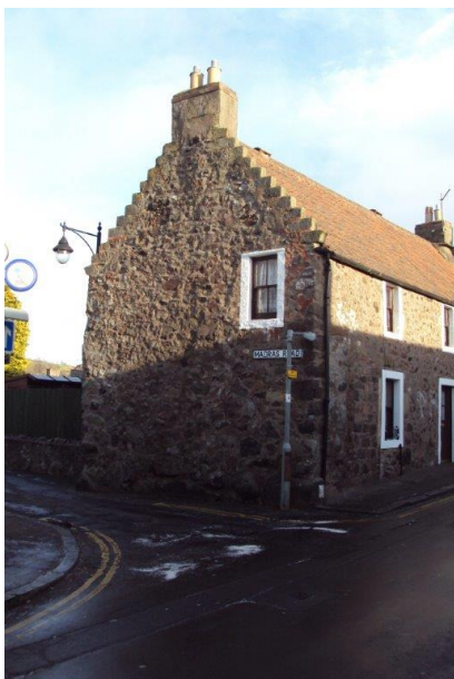
18 th century stepped gable, rubble masonry and pantiles.
