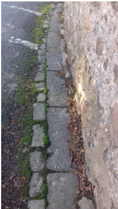
Surviving physical evidence for historic road surfacing and gutter detailing.
