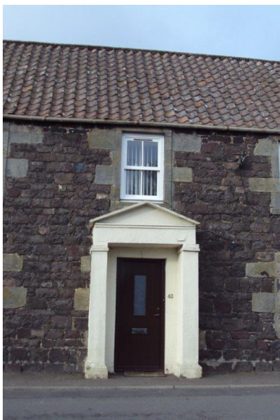
An example of the cumulative negative impact of the accumulation of historically inappropriate detailing: trickle vent; wide applied astragal and frame; glazed panel; letter box; door colour.
