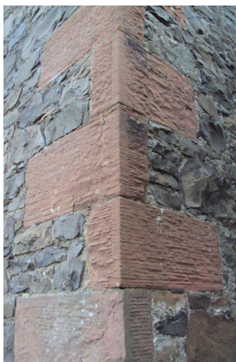
Example above right of whin laid to courses, using random sized and shaped units yet with ashlar tight joints, all exhibiting the highest craftsmanship. Red sandstone ashlar quoins (left) unusually, as most are plain, droved and broached.
