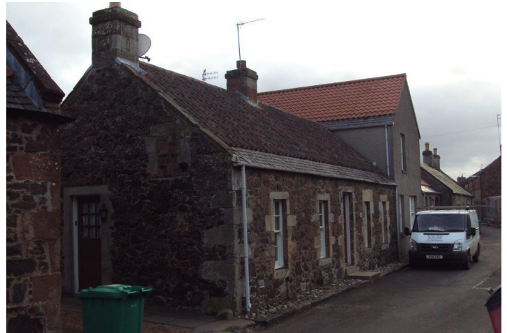
Note new development above with gable wall to road. Design includes pantiles and an over deep slate easing course but not a raised skew which is traditional.
