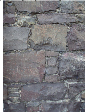
Whin masonry with the characteristic extensive use of pinnings (galleting) - cherry caulking (left) and ladder pinnings (right).
