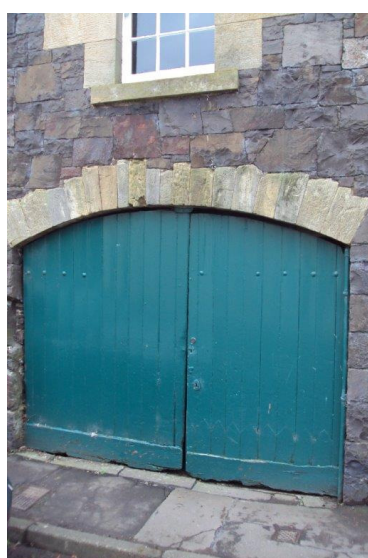
Contrasting examples of pend doors. Above left retains its original doors, the other has an inappropriate modern version.
