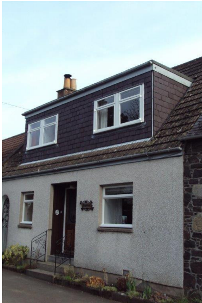
Examples above, below and right include: concrete roof tiles; roof windows; cement render; cement pointing; box dormers; modern style iron railings and gate; UPVc modern style windows and doors; plastic rainwater goods; cables; hanging baskets; trellis; carriage lamp; name sign; security camera/lighting; T.V aerials; vent pipes; meter box; modern plant varieties.
