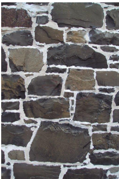
A fine example of cherry caulking and possibly original pointing mortar (above). Contrast this with inappropriate re-pointing (below), even though pinnings have been retained and the mortar is possibly lime based.
