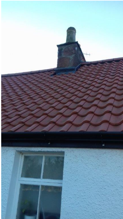
Although using clay pantiles, the modern detailing (lack of gaps or vertical edges) results in a roof of non-traditional character.
