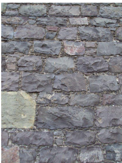
A fine example of cherry caulking and possibly original pointing mortar (above). Contrast this with inappropriate re-pointing (below), even though pinnings have been retained and the mortar is possibly lime based.
