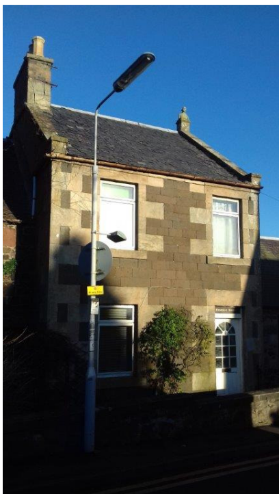
Example above of regular squared block, tightly jointed whin masonry.
