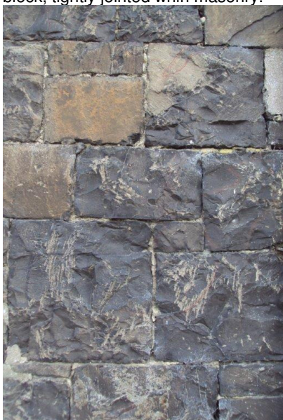
Snecked rubble masonry with its mixing of snecks, risers and levellers.
