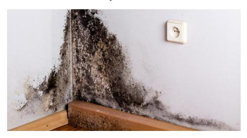
Penetrating damp is where water finds its way into the property from the outside. Penetrating damp is mainly down to poor maintenance of the building, this can be from leaking gutters, broken pipes or poor brickwork. If there are any gaps in doors or windows this can also lead to problems.
