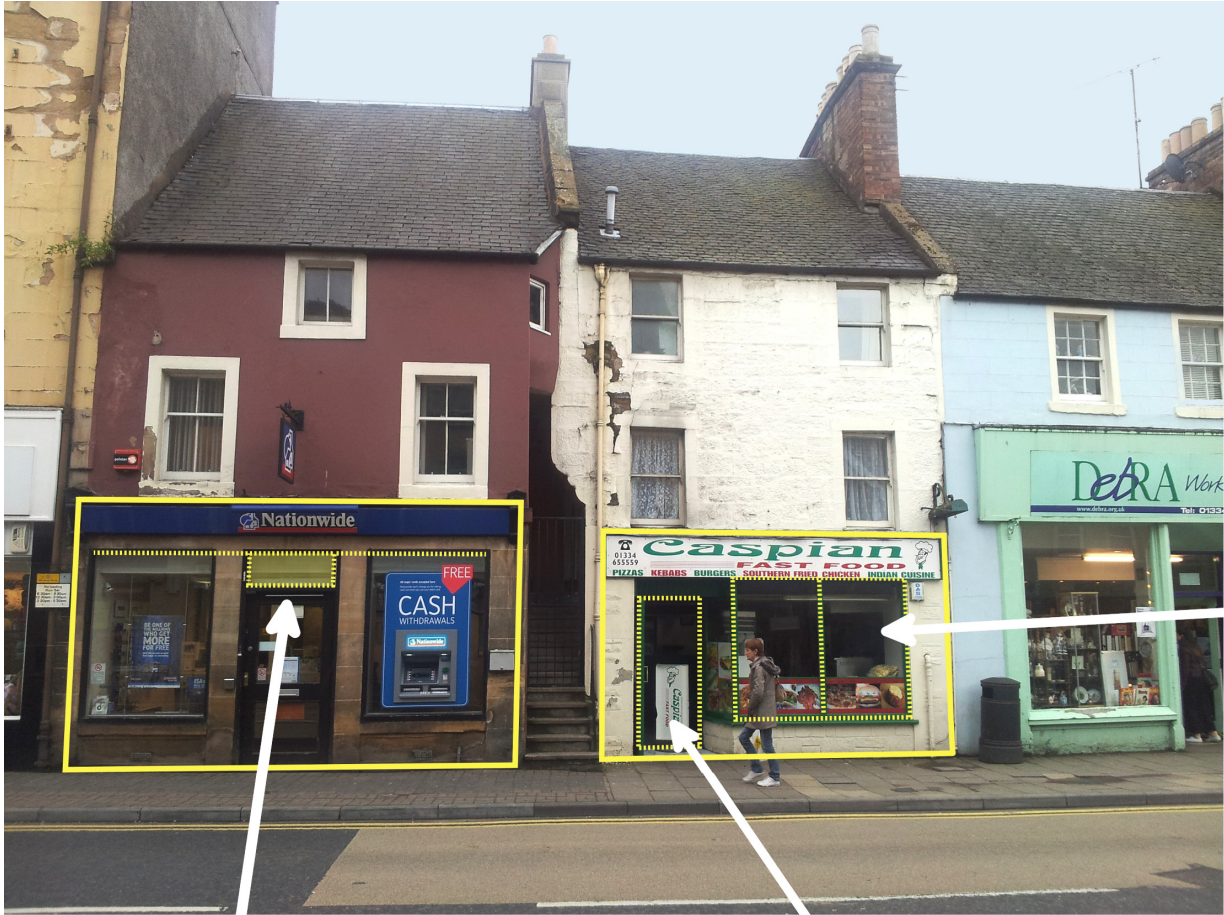
Windows above door, in line with window openings.
