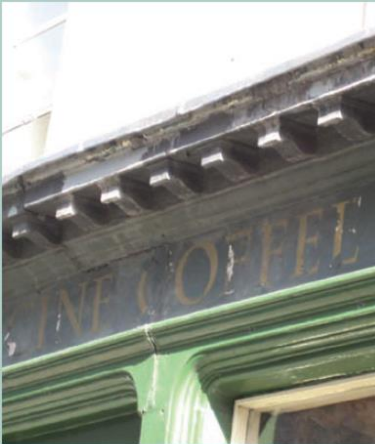
Removal of a modern fascia boards may reveal original details.
