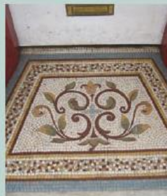
Example of the rich variety of traditional treatments of door recesses which can complement and enhance the character of the shop front.
