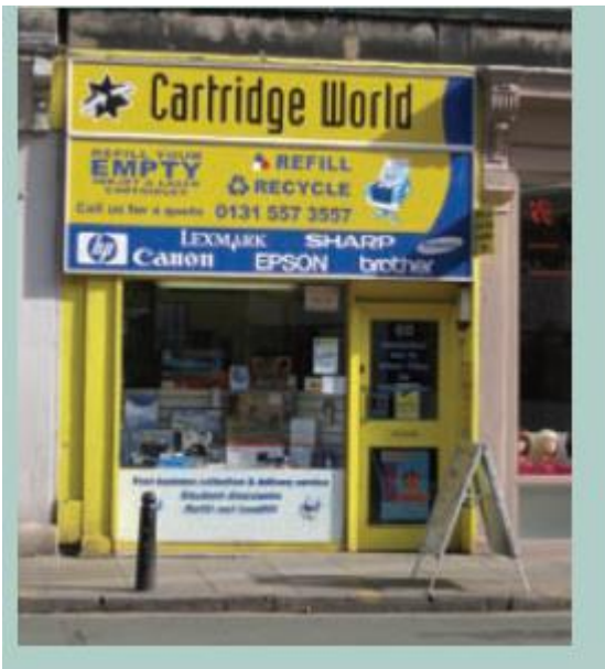
Example of inappropriate fascia board- excessively deep, obscured console brackets, cornices and pilasters.
