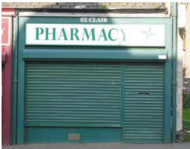
Example of unacceptable projecting box shutters
