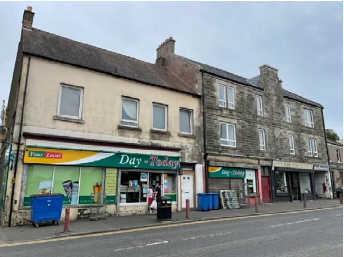
Street scape at the North end outside the bingo hall
