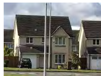
3.4.3 Suburban Housing (Dalgety Bay 2022)
