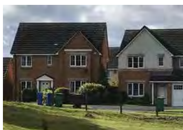
3.4.2 Suburban Housing (Dalgety Bay 2022)
