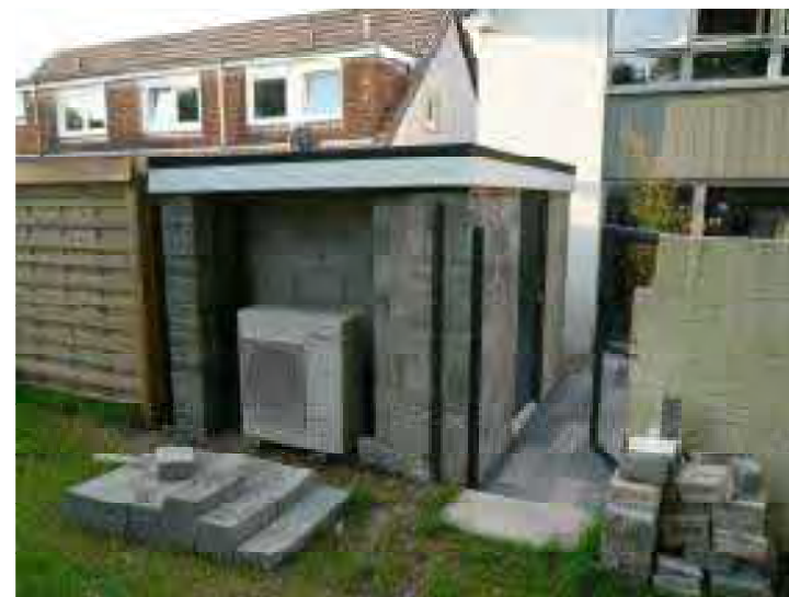
Photo 3.0: 41 Learmonth Place – new garden shed and heat pump (2021).
