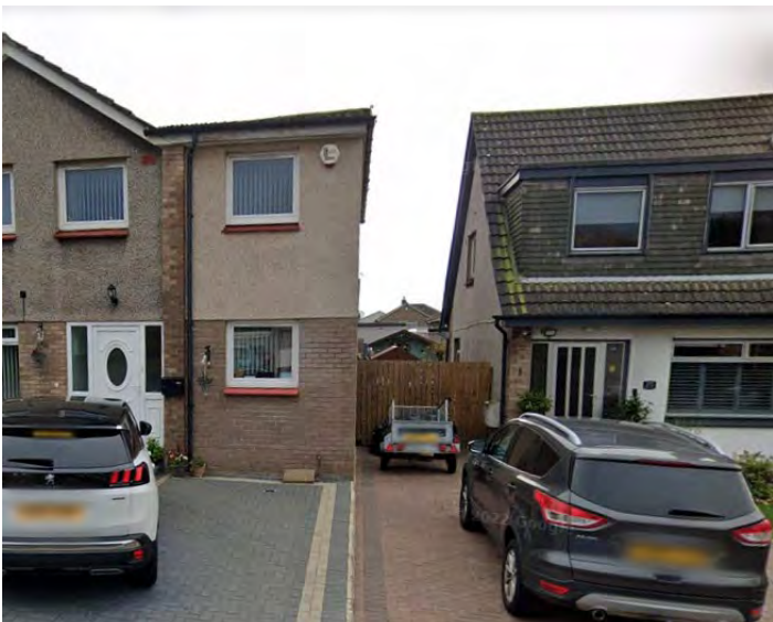
28 Beech Grove (again a two storey in close proximity to neighbouring kitchen windows etc all approved by Fife Council)
