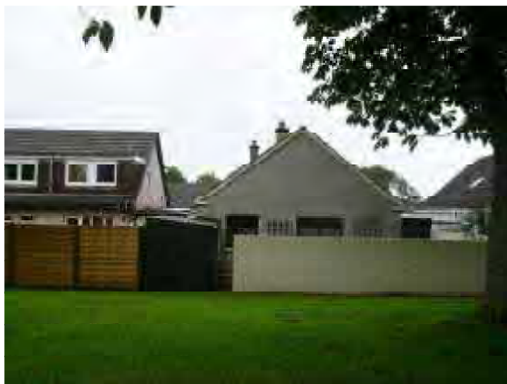
Photo 2.0: 41 Learmonth Place – original house and garden shed (2019).
