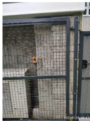
Photos 3 & 4: The welded metal frame
