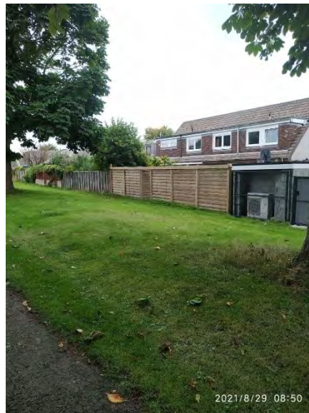
Photos 11 & 12: The ASHP and its plantroom are immediately obvious
