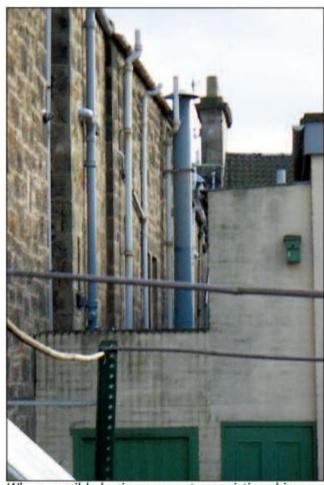
Where possible, businesses must use existing chimney flues to remove cooking smells. Where this is not possible discreetly located flues in rear elevations may be acceptable
