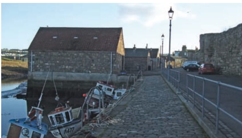
Traditional quayside warehouse forms on Balfour Place with dominant gables, simple lines and strong boundaries
