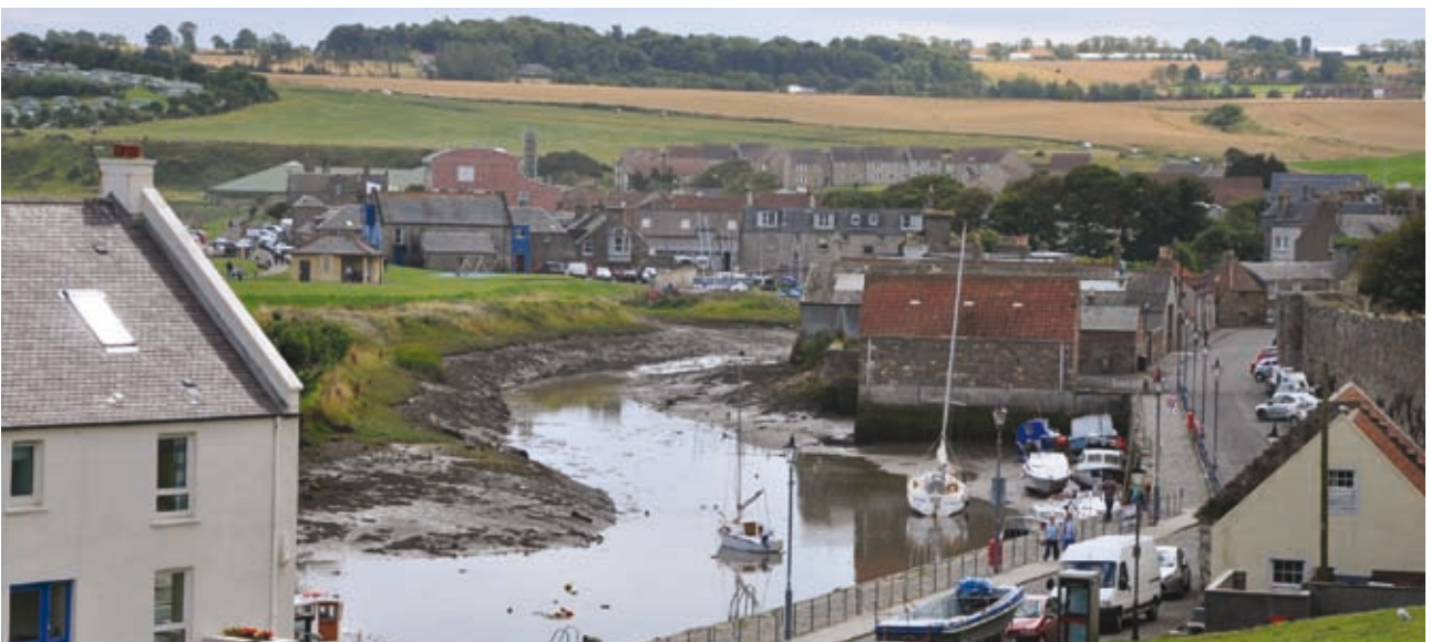
View 11 – From Fife Coastal Path over Kirk Hill. As View 10. Comparison of both reveals the importance of building height and massing in the Framework Area.
