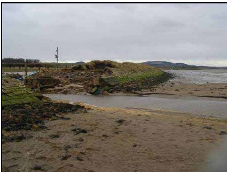
Figure 7: Storm Damage and Flooding in March 2010 at the South Bank of the Eden Estuary (Former Railway Embankment). Managed Realignment is the preferred policy, recognising the aims of the Eden Estuary SPA, SAC, Ramsar and SSSI designations.
