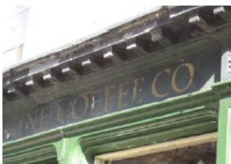
Example of acceptable hand written lettering sign (above) and national multiple sign adapted to fit fascia (left).
