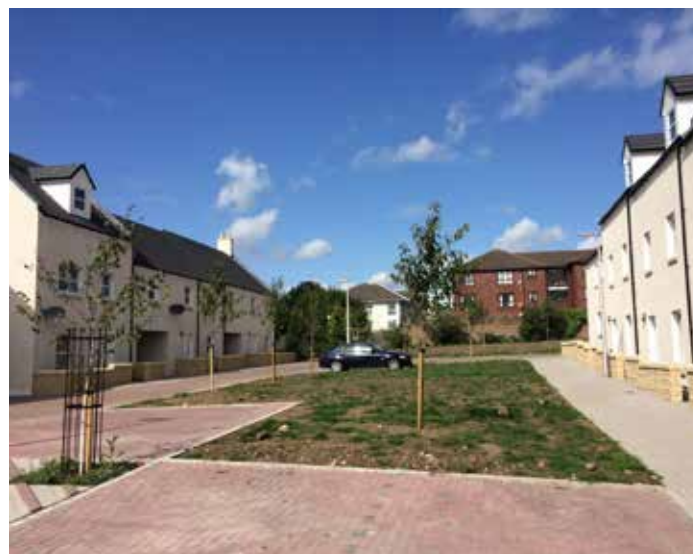
Greenspace unuseable: Not seeded & large stones
