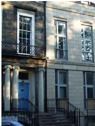
Eaves, storey heights and string courses consistent with adjacent. Windows/ balconies sizes and proportions reflect adjacent, but style and materials are contemporary
