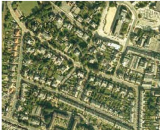
This image shows how the streets are connected, making it easier to move around or through, with a choice of routes - making the area 'permeable'.
