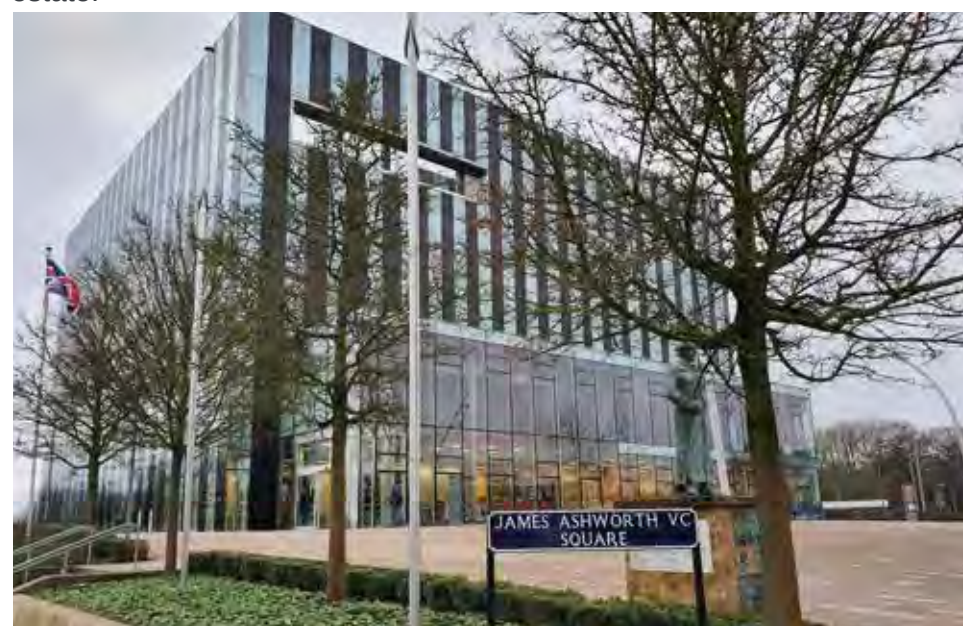
Figure 54 - Corby Cube – multi-functional public sector hub
