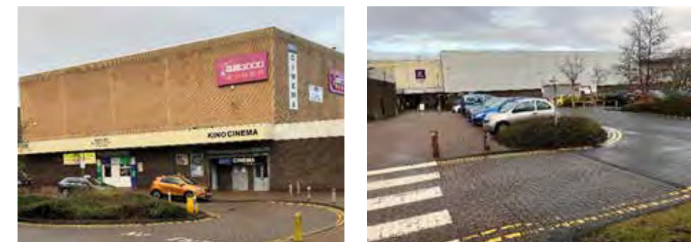
Figure 34 – Church Street entertainment complex, Kino Cinema, Club 3000 Bingo, pub and restaurant
