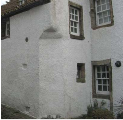
Chamfered corner on Mid Causeway
