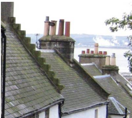
Crowsteps and skews at Tanhouse Brae seen against the smoke of Grangemouth.
