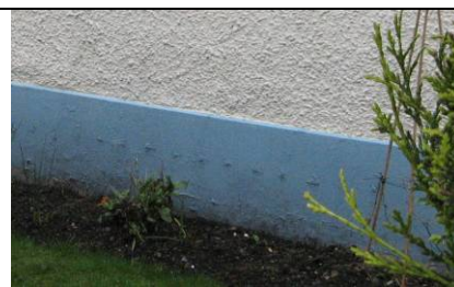
Injected damp-proofing
