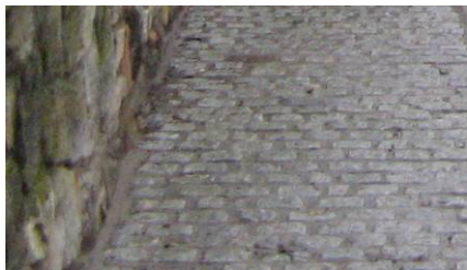
Pavement setts laid in a traditional manner on Low Causeway
