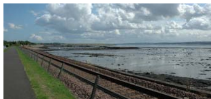
View across the railway towards the foreshore.
