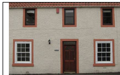
Replacement windows, uPVC, set far forward in the opening
