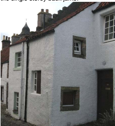
Rowanbank, Back Causeway, showing the front jamb, formed with a catslide roof.
