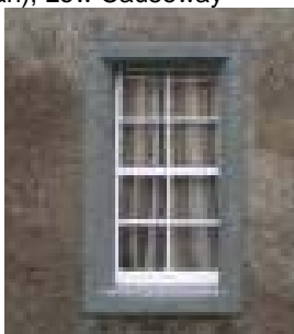
close-up of window of House (D Morgan)
