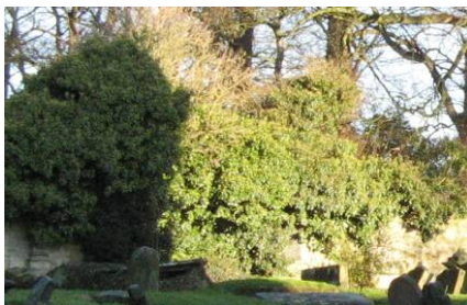
Heavy vegetation growing on one of the (listed) boundary walls of the Abbey graveyard
