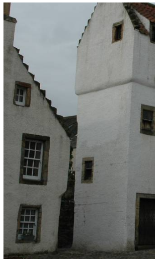
Left: Jettied upper level at The Study, chamfered corner on 6 The Cross. Right: jettied upper level at 7 Mid Causeway.
