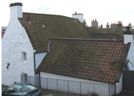
Rowanbank, Back Causeway, showing the single storey back jamb.
