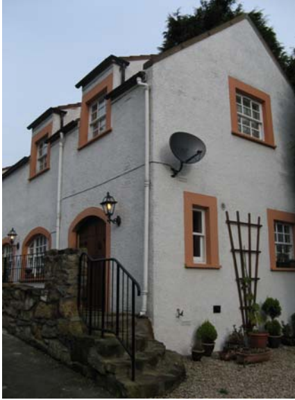
This house on Mid Causeway does not match traditional detailing in several aspects – treatment of the gable, window and door openings and margins, colour, external fixtures, treatment of curtilage.
