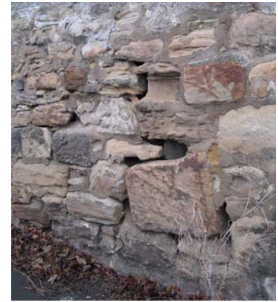
Left: view inside the building. Right: decayed rubble wall.
