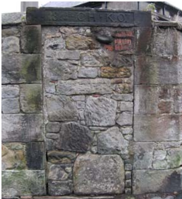
Wall at corner of Back Lane and Erskine Brae, with inscribed lintel, probably from Clifton House (now demolished).
