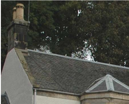
Undercliff, West Green, has several typical elements of roof detailing.
