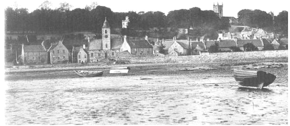
View from Culross Pier, showing the village before the reclaiming at Sandhaven. (Beveridge, frontispiece)
