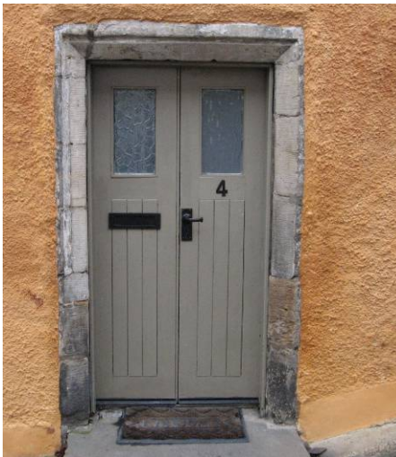
A typical double-leaf timber door at 4 Tanhouse Brae
